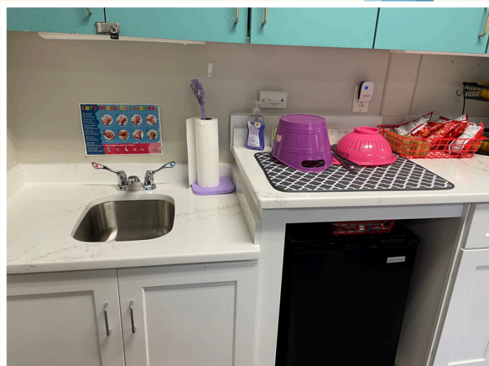
Installed new granite countertop, sink, cabinets and refridgator for Classroom 11 at our Quinn Center
